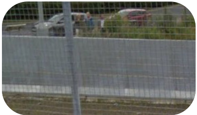
VGSP-04 A 1800mm-high steel post and vertical infill solution with posts installed at 2.0m centres. Solid sheeting is affixed to the pedestrian side of the system.
