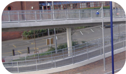
VGSP-01 A 1150mm-high steel post and vertical infill solution with posts installed at 2.0m centres.
